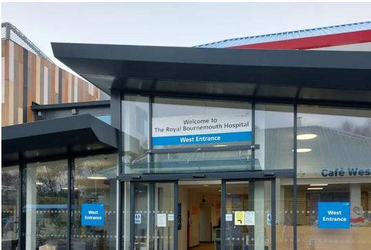
An example of a hospital entrance with automatic doors and signs.
